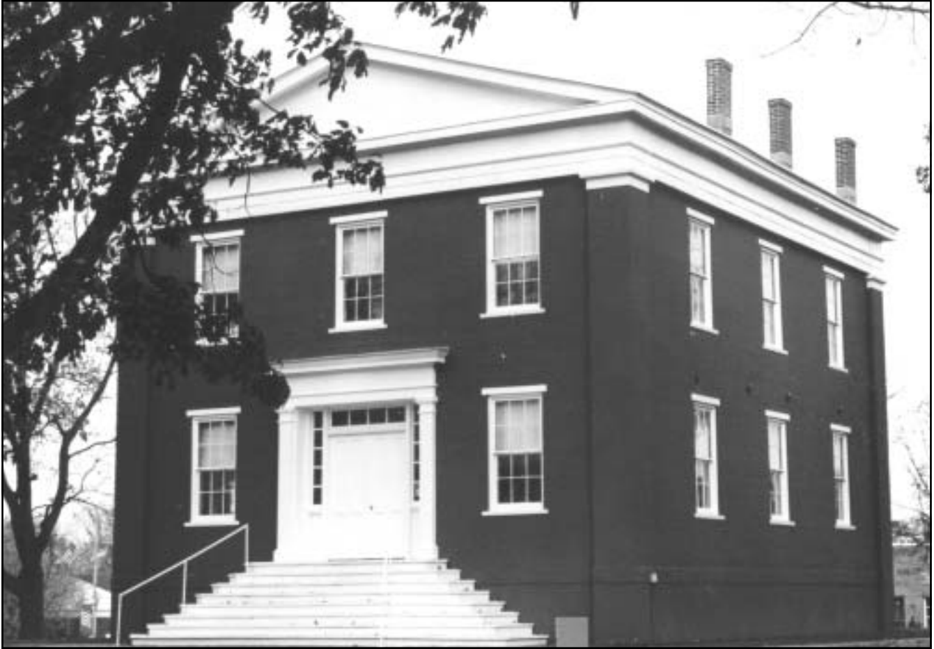
Figure 7. Logan County Courthouse, Mt. Pulaski, Illinois, 1848-1854. Photo courtesy of The Papers of Abraham Lincoln .
